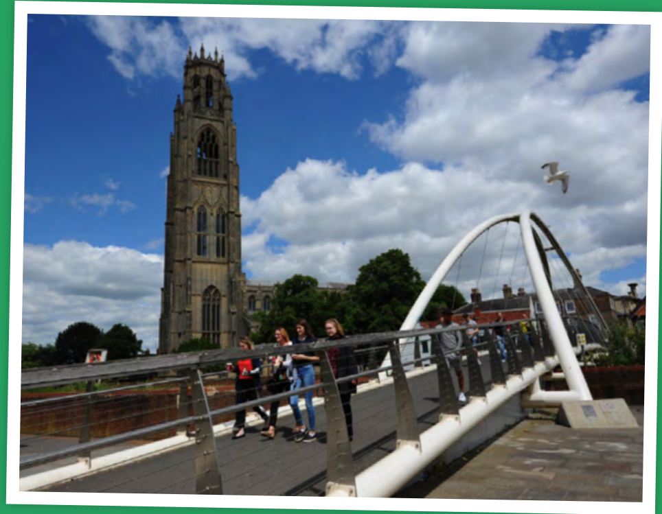
St Botolphs bridge, Boston 2019 © Courtesy of Boston Borough Council
