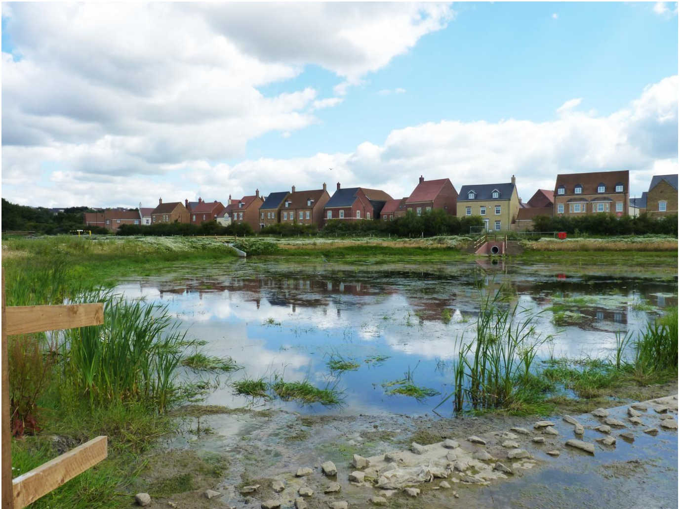
Flood alleviation. Wichelstowe, Swindon © Arup
